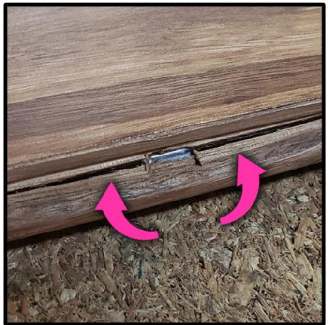
Cleat properly driven and some splitting
